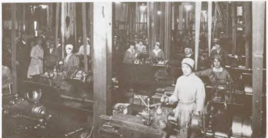
1918. Machine Shop, Telegraph Works.
