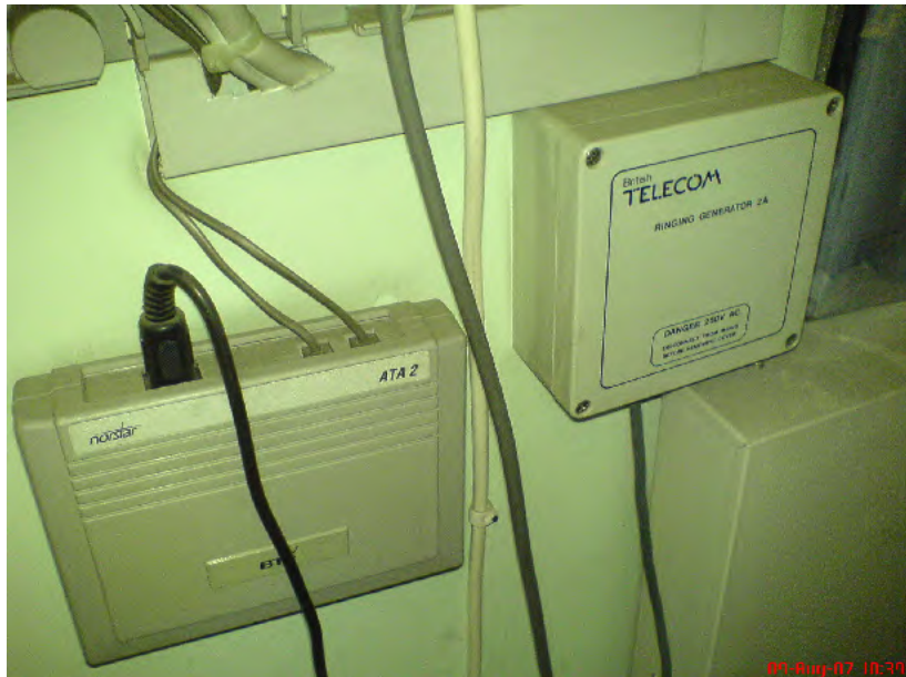
Norstar ATA module on the left and an external bell ringer on the right
