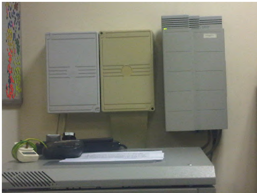
Norstar Compact plus system with CPU card and trunk cards inside the cover
