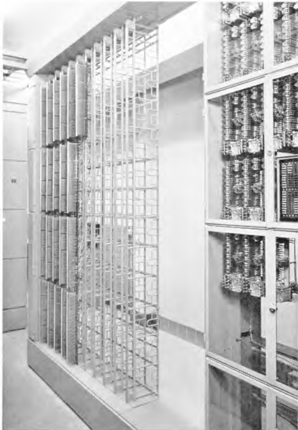
intermediate distribution frame
