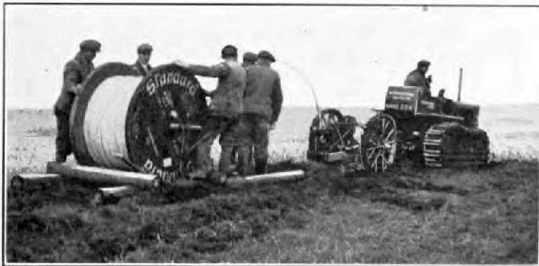
FIG. 3.—CABLE-LAYING WITH MOLEDRAINER AND SLEDGE.
