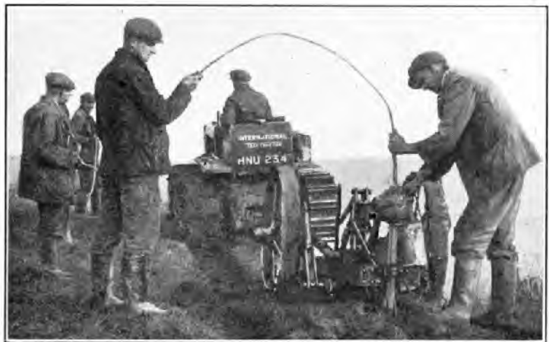
FIG. 2.—CABLE-LAYING WITH MOLEDRAINER.
