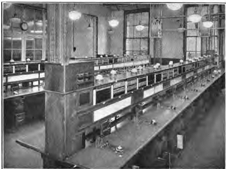
FIG. 1.—THE PHONOGRAM SWITCHROOM AT NEWCASTLE, EQUIPPED WITH DOUBLE-TIER ANCILLIARY SWITCHBOARDS.
