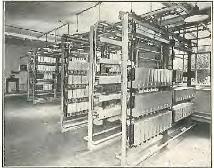
FIG. 1.—TYPICAL 500-LINE INSTALLATION OF P.A.B.X. No. 3.
