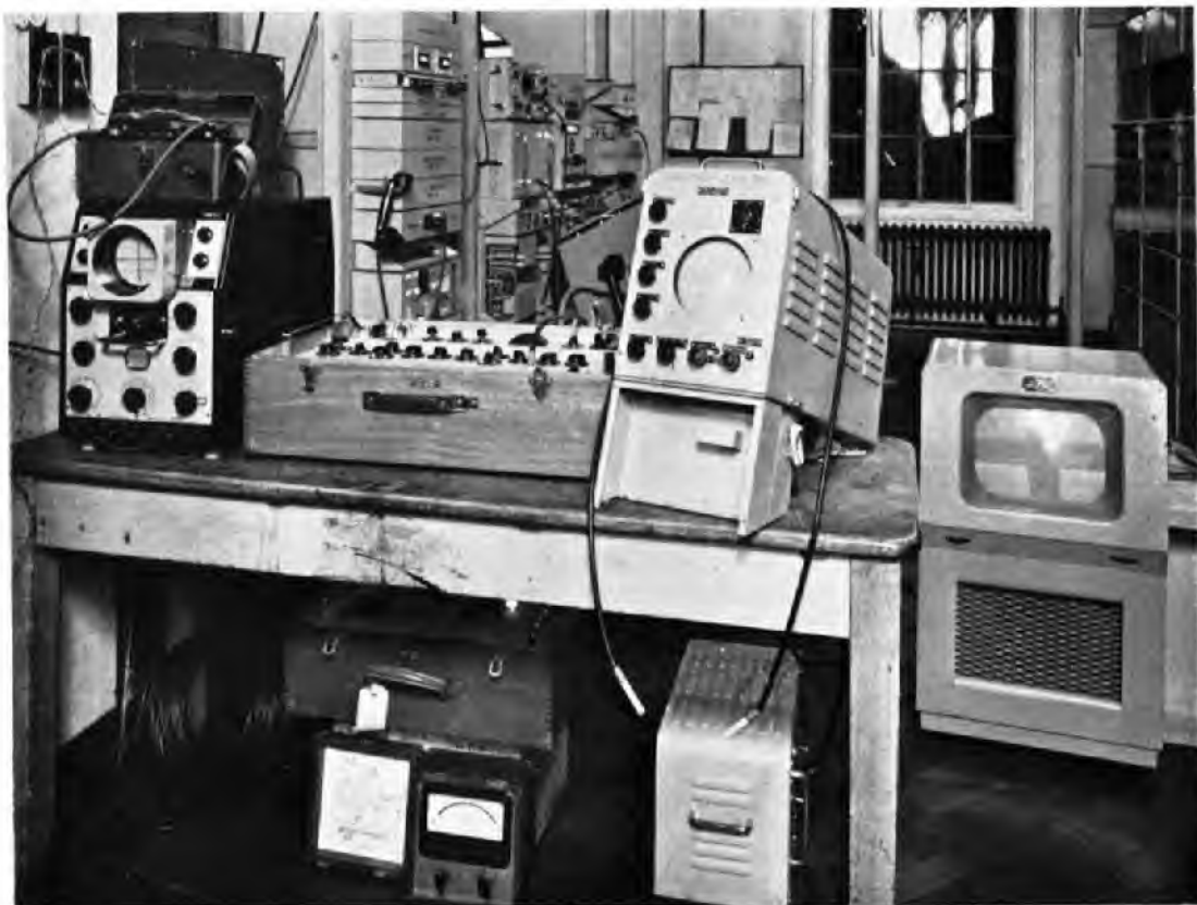
Fig. 6: Terminal video repeater and injection equipment at Cardiff repeater station
