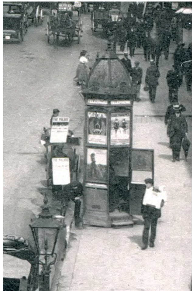
Figure 2. The westernmost of the three former Street Syndicate Ltd kiosks in High Holborn, c. 1903.
