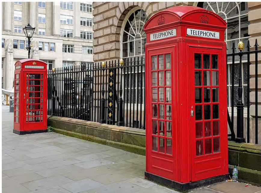
Figure 16. Grade II Listed K2 kiosk (Listing No. 1262058) on Exchange Street West, Liverpool (outside Liverpool Town Hall) alongside a K6. Sadly, the reproduction signage on the K2 has been very poorly implemented (photograph taken 15 September 2018).
