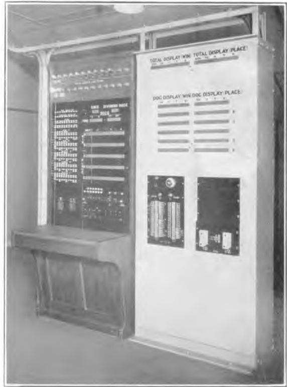
Glasgow (White City) Greyhound Racecourse— Control Switchboard and Miniature Indicator
