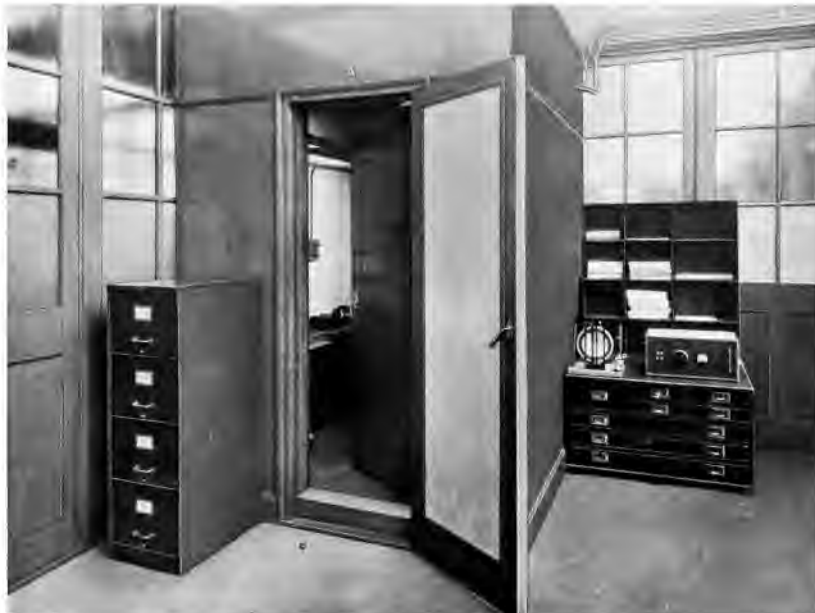
Fig. 3.—Typical silence cabinet.
