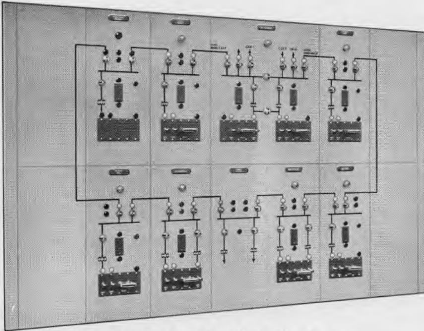
Fig. 4.—Supervisory Control Panel showing Mimic Diagram.
