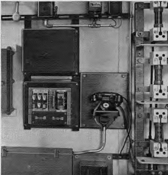
Fig. 2.—Substation Supervisory Control Cabinets.
