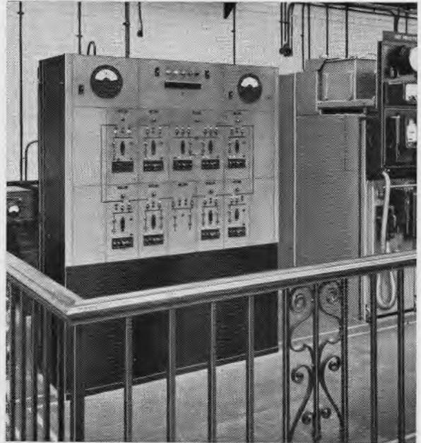
Fig. 3.—Supervisory Control Cubicle at Power Station.
