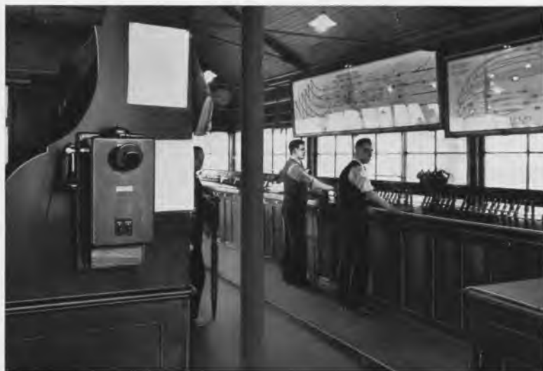
Fig. 5.—Selective ringing telephone in signal cabin.
