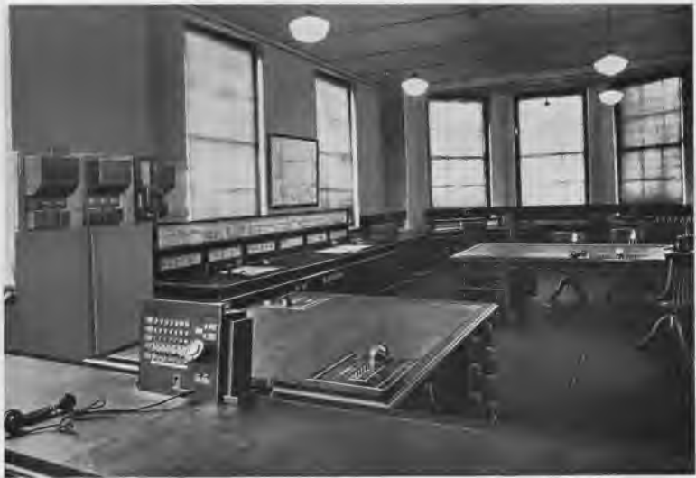
Fig. 1.—Control Room, Darlington.
