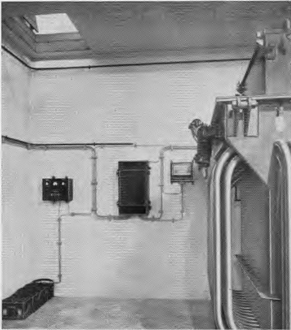
Fig. 4.—Remote supervisory control apparatus at Avenue Mews substation.
