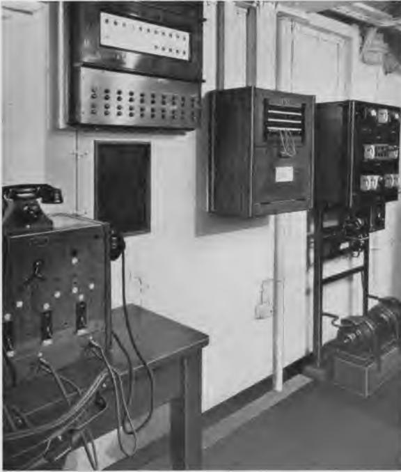
Fig. 5.—Service clerks' cabinet, stewards' line coupling cabinet and power plant.
