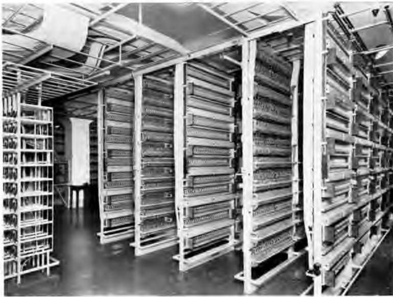
Fig. 6.—Uniselector racks.
