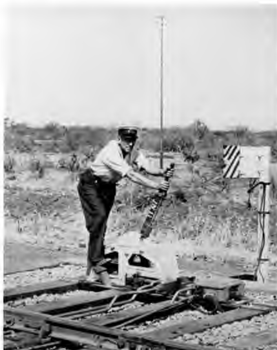
Fig. 8.—Operation of main-line points at end of loop.
