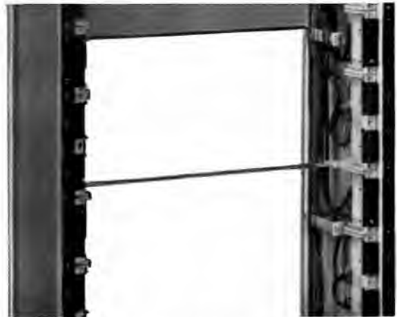
Fig. 9.—A section of the framework of an unequipped rack, showing the guides on which the panels slide into place.
