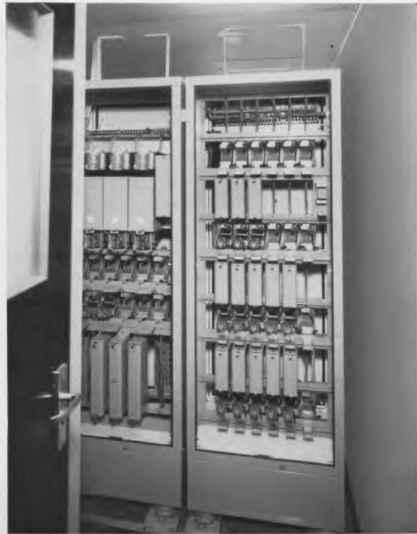
Fig. 8.—Automatic telephone exchange on “Oriana”
