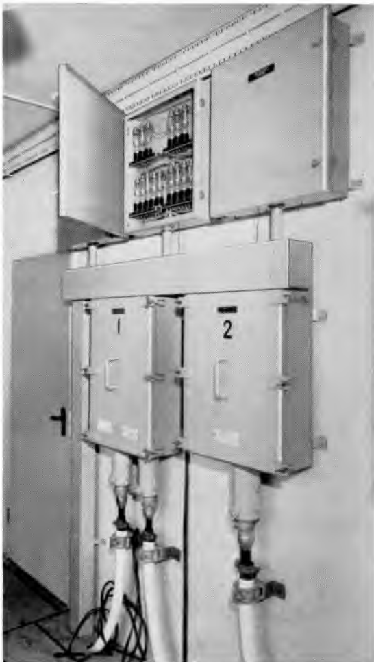
Fig. 7.—Line-protection equipment.
