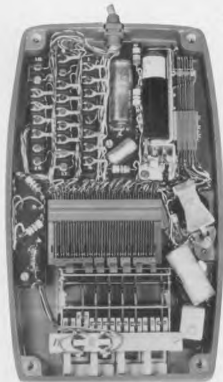
Fig. 4.—Internal view of plinth.
