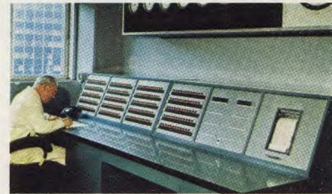
Production Recording & Control Console
